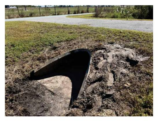
Photo 3: MES2 (Sediment Removed and Filled Depression to Right of Pipe)
